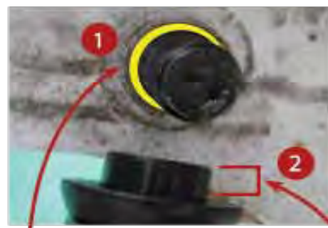
1) YELLOW HIGHLIGHT shows void between stud and stud hole. 2) Skirted Nut fills void between stud and hole.
